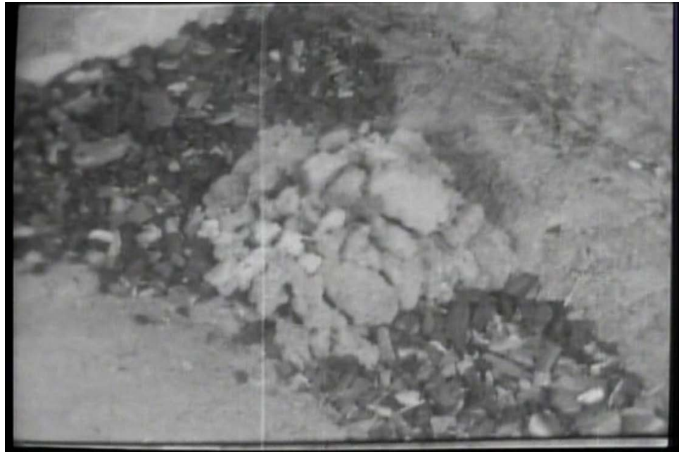
Fig.4 Process 1 Construction of steel blocks like tunnel 6,9)
